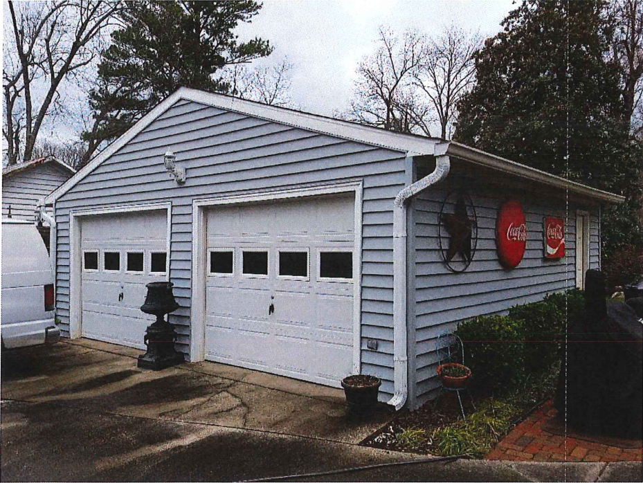
Existing Garage: View from House Back Door
